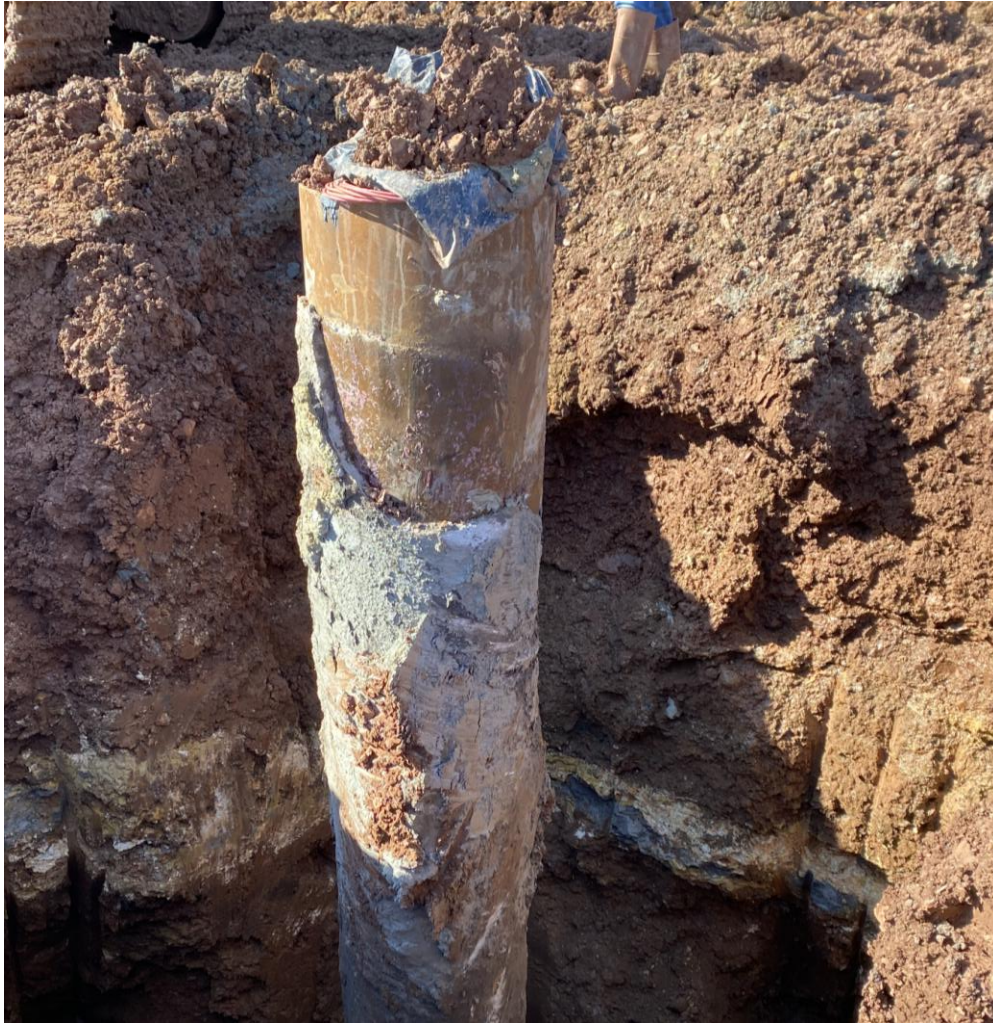
A pile with the casing extended, then excavated
